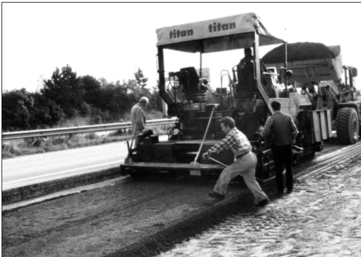
Fig. 8: Road construction with ash for the bearing layer
