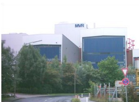
View of MVR: MVR is located right the banks of the River Elbe in the Port of Hamburg.
